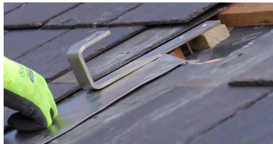
Products and processes have been specifically developed to securely fit panels to existing roofs. Example shows a stainless steel roof hook being mounted to a slate roof. (Source: Schletter installation video)
