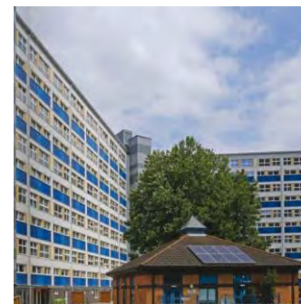
Wilmcote House, Plymouth (Source: ECD Architects)
