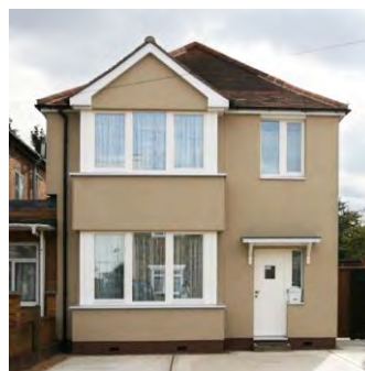
Grove Road, London (Source: Bere Architects)
