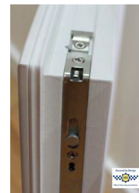
Multi-point locking mechanism (Source: Sashed)
