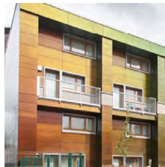
Ernley Close, Manchester (Source: 2e Architects)
