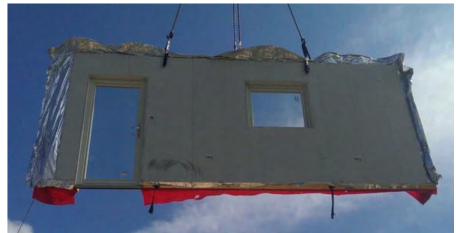
A closed-panel timber frame, manufactured off-site with insulation, window and door frame included (Source: Vision Development).
