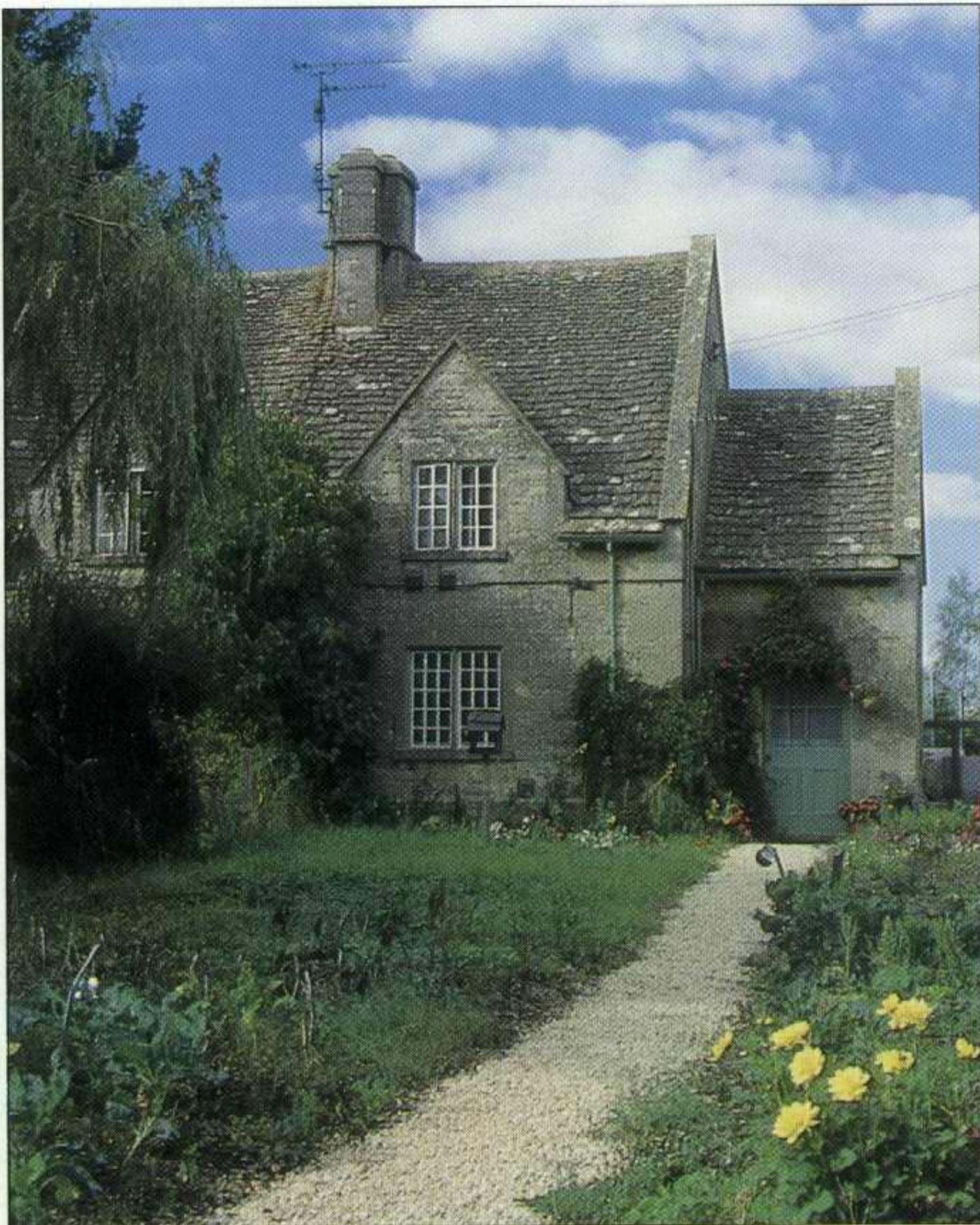
Another typical and highly attractive estate cottage, with the visual proportions, window forms, and Cotswold stone slate roof that are to be encouraged in future building design.
