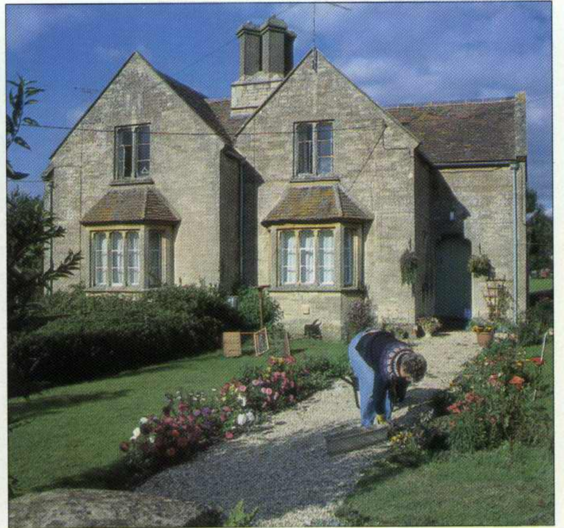
The estate cottages built in the nineteenth century are a feature of the village, with their bold windows and porches, and attractive well-maintained gardens adjoining the main street. This pair of cottages is more elaborate than most.
