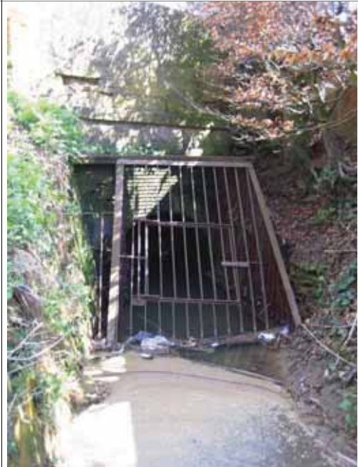
Photograph - Existing trash screen on the inlet to the culvert in Queen Victoria’s Garden (12)
