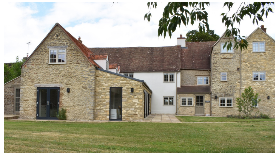
Rural properties with multiple phases of construction
