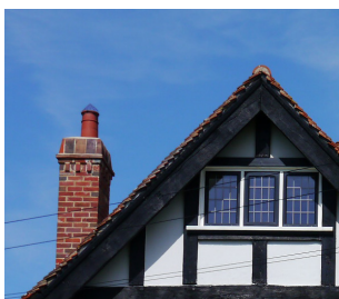
Gable ended roof
