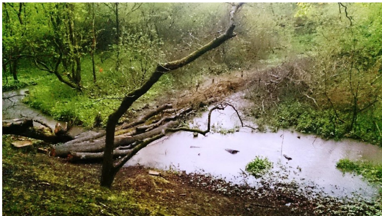
Figure 9.6: Photograph of leaky dams at Black Brook.
