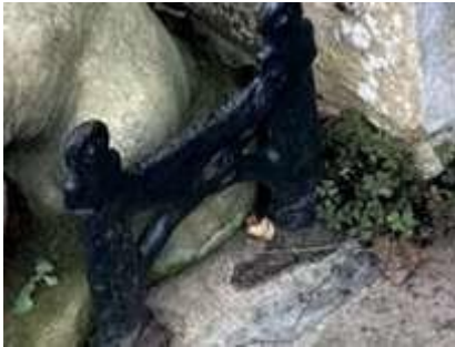
Ivy House, High Street, GL55 6AG
