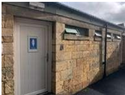
Toilets at The Old Police Station The Old Police Station courtyard, The Old Police Station, High Street, GL55 6HB
