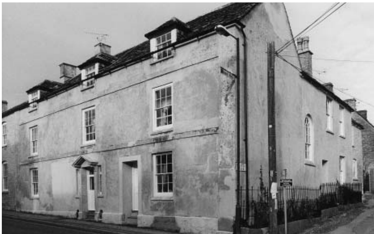
This fine group of 18 th Century buildings, which incorporates the former Reading Room, are constructed of natural stone and coated with a lime render and limewash, finishes which are characteristic of this part of the Cotswolds.
