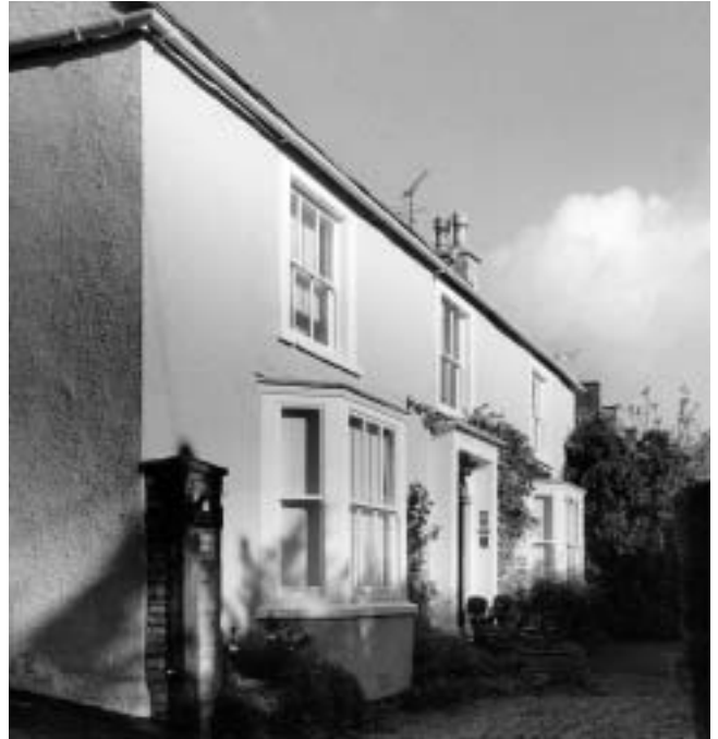
Roughcast render is the characteristic finish of many of the buildings in Didmarton, as seen on the grade II listed Old Rectory.
