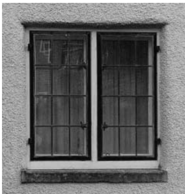
Leaded, wrought-iron casements set in timber frames are a particular feature of the village.
