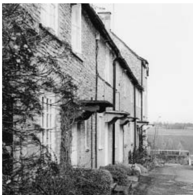
The row of cottages in Chapel Walk still retain their stone porch canopies.
