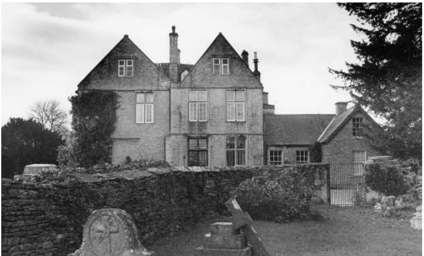
The Manor House, a grade II listed building, dates from the late 16th and 17th Centuries and was re-fenestrated in the 18th Century and enlarged in the 19th Century.
