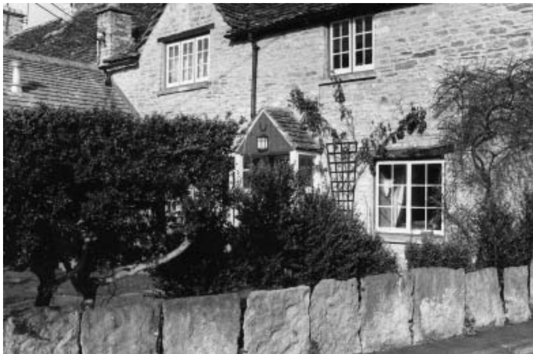
School Lane begins with a very distinctive boundary treatment formed from large stone slates. The rear elevation of Highnam Cottages reveal themselves to be very well preserved examples of traditional cottage architecture.
