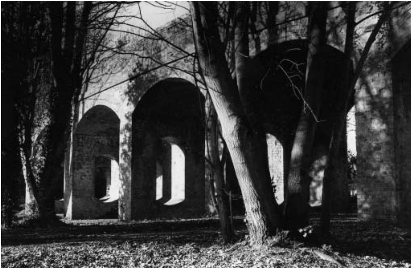
A disused railway bridge carries the lane out of the village at the eastern extremity of the Conservation Area. On top it provides a rare elevated platform for viewing the expanse of meadowland to the north. From below its magnificent structure of brick arches sets a quite contrasting intimate scene.
