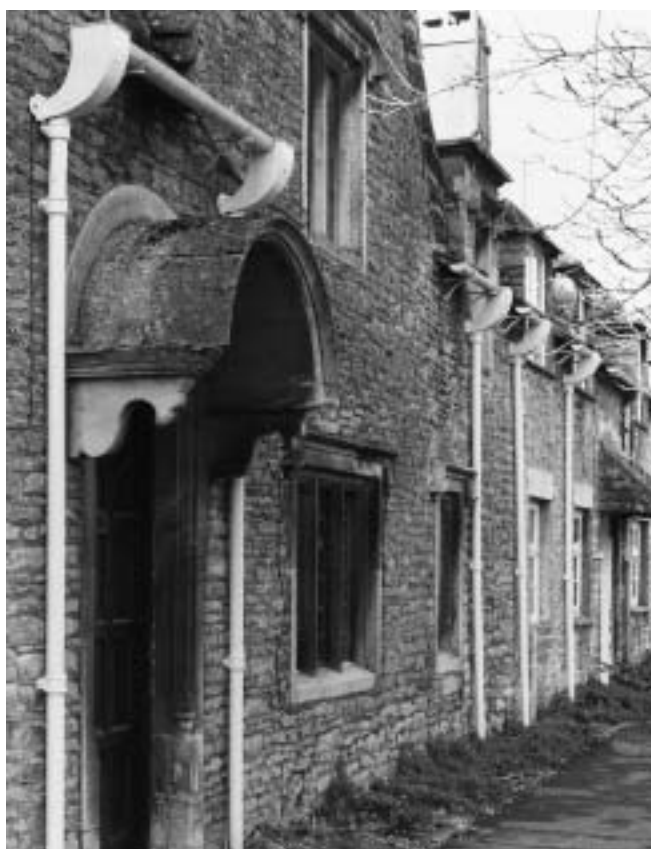
The distinctive architectural details and painted cast iron rainwater hoppers of the cottages on the west side of Silver Street help to enliven the scene.
