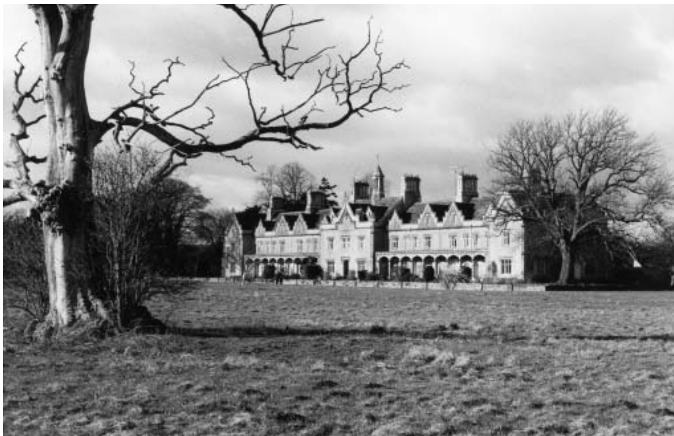
Edwards College is an impressive building of the Gothic style which fronts an expanse of open fields which eventually lead south-east to Chapter Manor. Although not publicly accessible, this is a very important open space within the Conservation Area.
