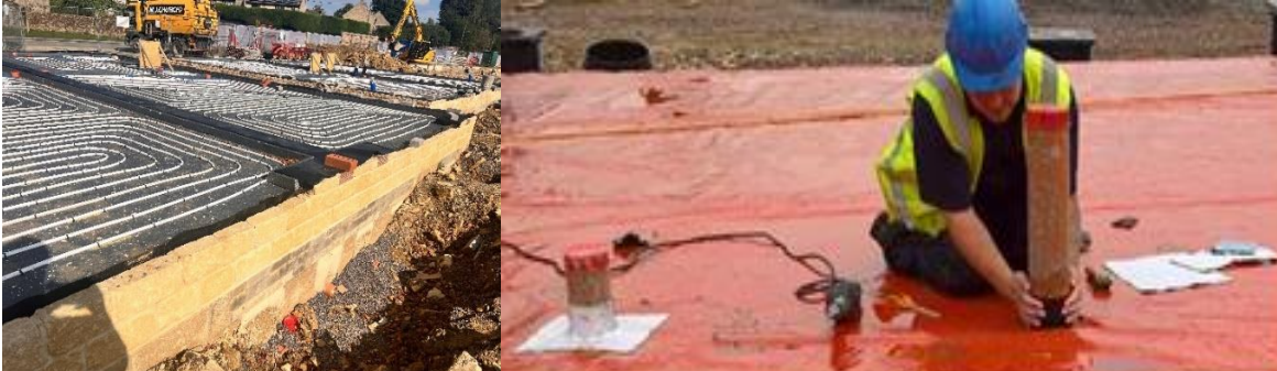
FIGUREs 5&6 Remedial works undertaken as per the site investigation recommendation – installed gas-resistant membrane on housing foundations (left, 5); installation of a seal around pipework penetration of the gas membrane (right, 6)
