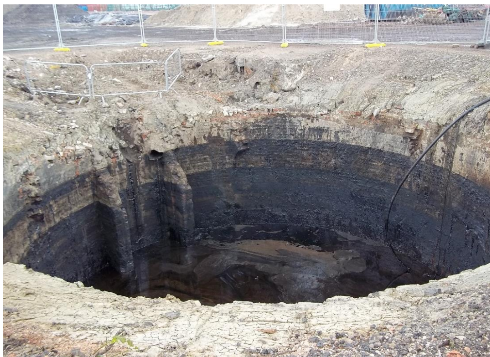
FIGURE 4 Removing tar from a disused gasholder
