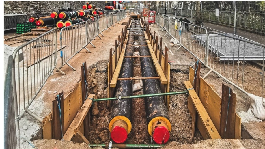
Heat networks relies on distribution pipes. Medium/high distribution temperatures and long pipes will have high distribution losses (Image source: Vital Energi)
