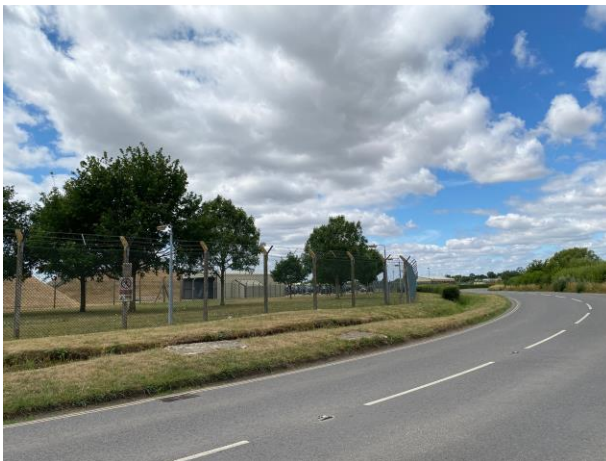
RAF base with fencing and buildings within a semi-rural context.
