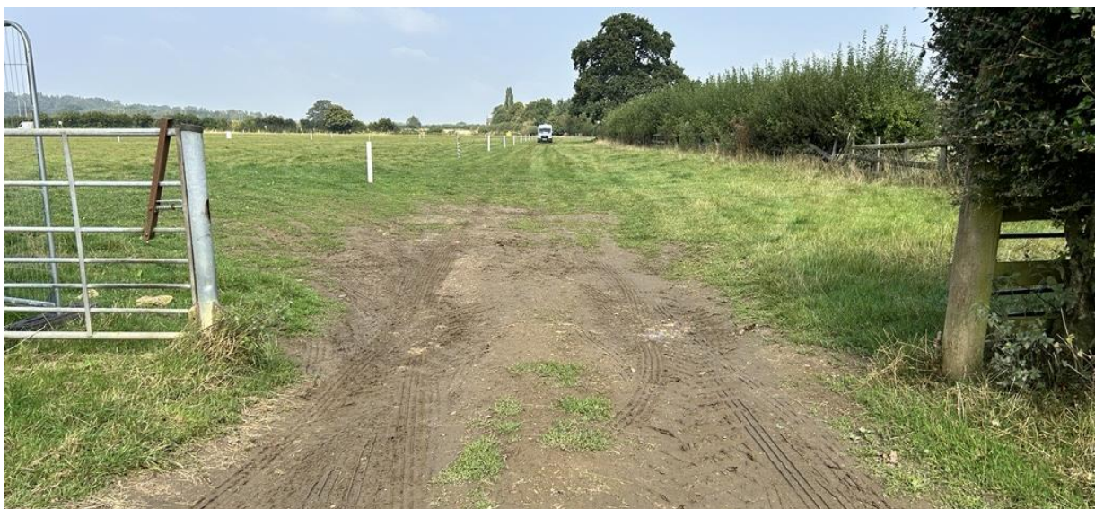
Image: The entrance/exit to the blue badge car park showing ground conditions.
