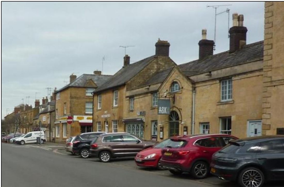
Figure 2-22: Parking overhanging carriageway
