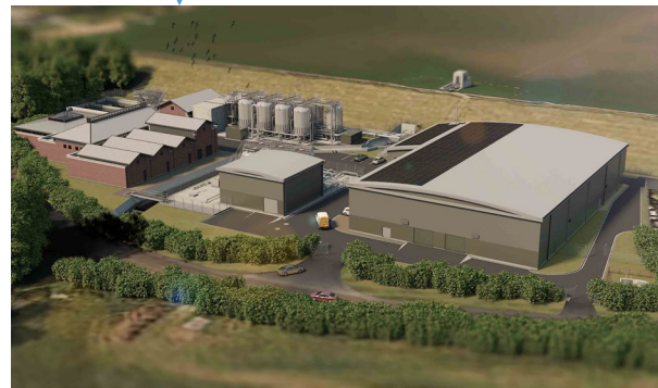
Treatment and distribution
