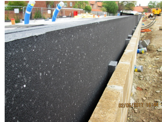
Good examples of insulation installed on site, showing methods to eliminate gaps (wedging and overfilling). Left: Goldsmith street © Etude, Right: © Green building store.
