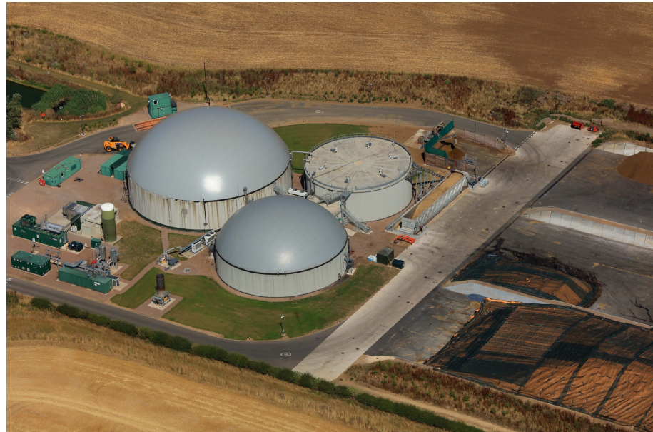
Typical anaerobic digestion facility. Biogas can be produced from waste and used to generate electricity. © The association for renewable energy and clean technology.
