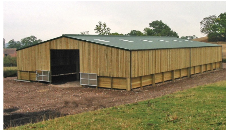
Agricultural and light industrial buildings offer a great opportunity for energy generation through PVs.
